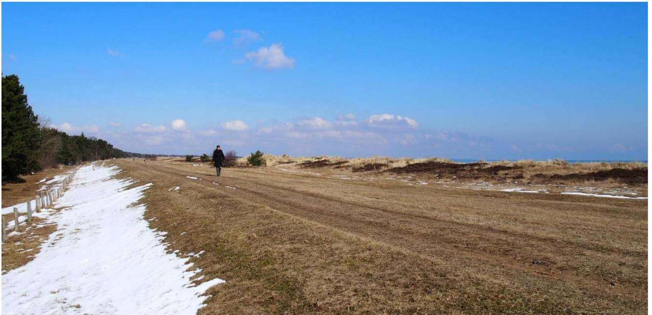
*Figure 5. The 17 km dike along the southern part of the east coast of Falster was constructed rapidly after the 1872 storm surge, and was finished in its present form already in 1875. During the following 138+ years a ridge of sizeable sand dunes has accumulated on the coastal side of the dike (to the east). The dike is seen in the foreground, and the sand dunes to the right. View towards NNE. March 15, 2013.*
